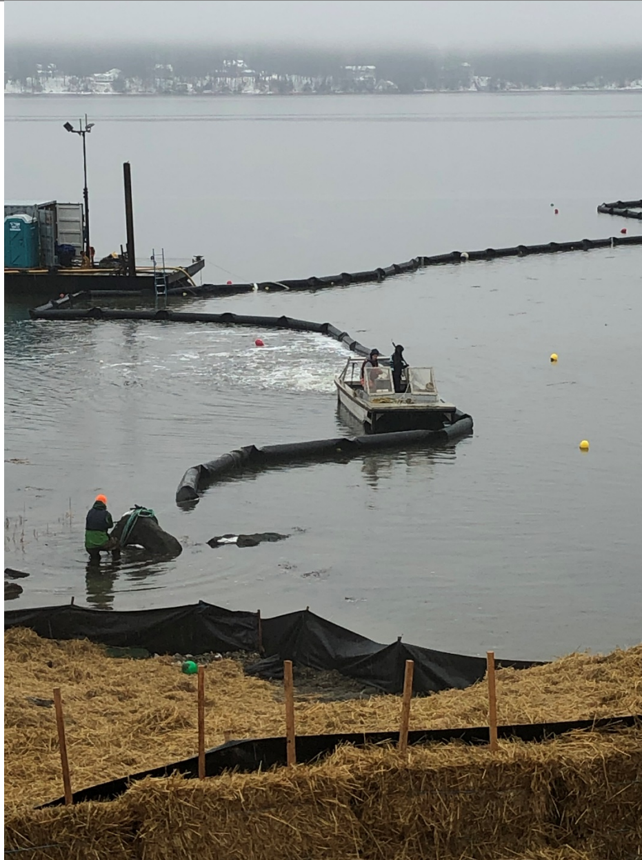
View from Getchell Property, Durham, NH showing Mackwork Env staff adjusting northern end of the turbidity barrier on the west side of Little Bay because it moved, or was moved, offshore resulting in a gap at the shoreline (12-9-19).
